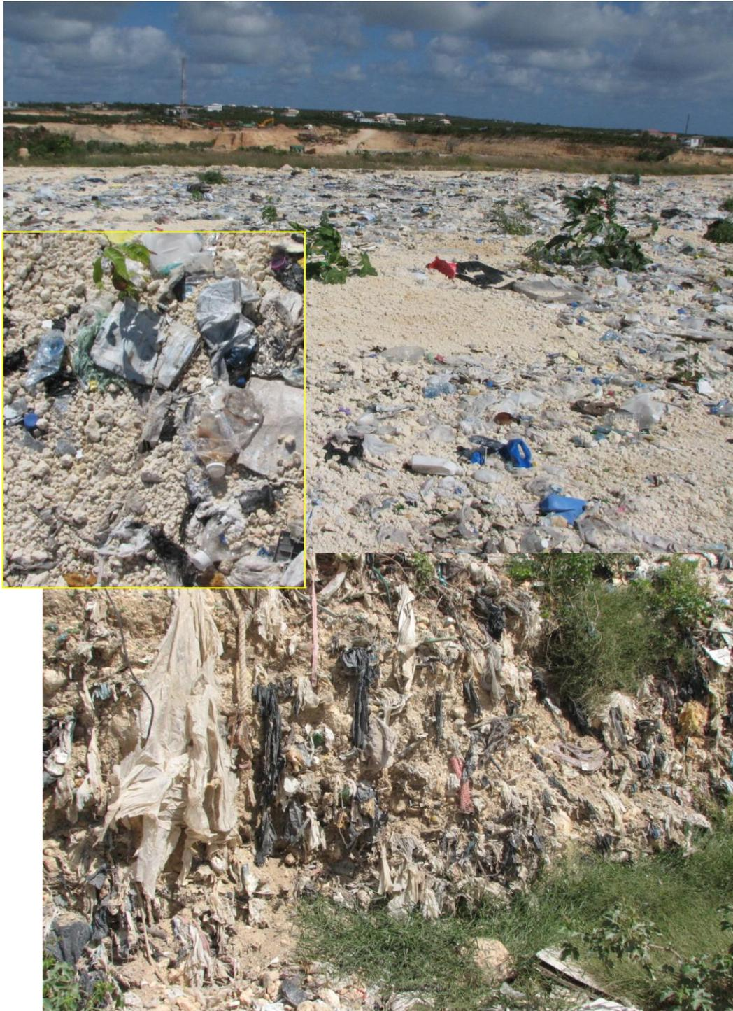
*Anguilla dump after covering with crushed marl. Note the coarse cover and difficulty covering plastic with the rock.*
